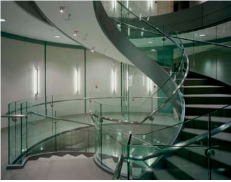
Curved tempered glass railing Office Building, Washington, D.C.
